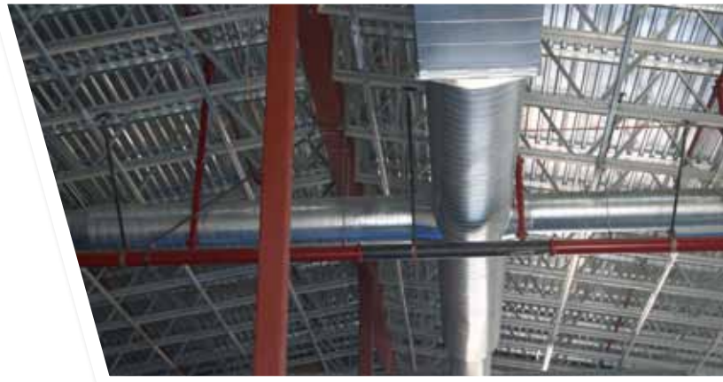
A knuckle boom was needed to thread Burch's men through the red iron and subsequently install the bottom chord bracing.
