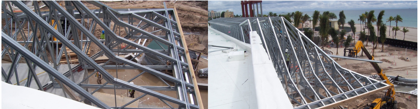
A cantilevered truss design, reflecting the shape of a Polynesian-style roof, incorporates many TrusSteel Cold-Formed Steel Truss System sections.
